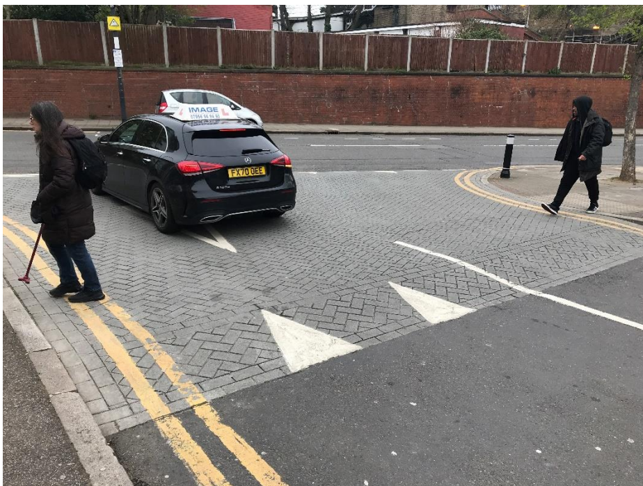
An example of a change of surface for people to walk across a junction. Wanstead, London
